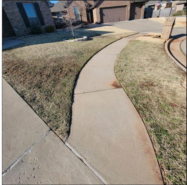
2.4 Item 2 (Picture) Walkway
