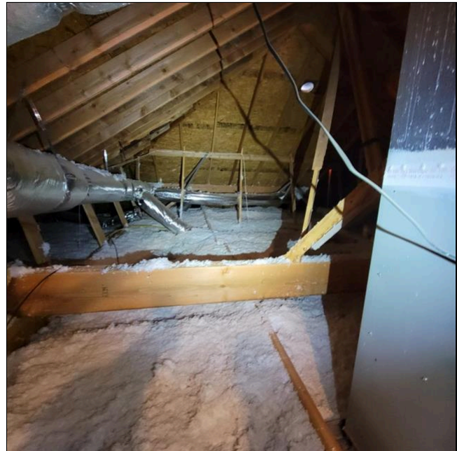
1.5 Item 2 (Picture) Roof Structure
